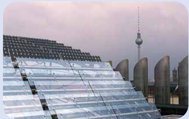
Three quarters of new buildings should have solar panels
